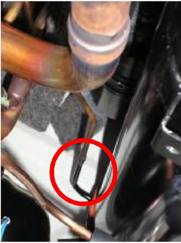
Refit the heat exchanger drainage channel
