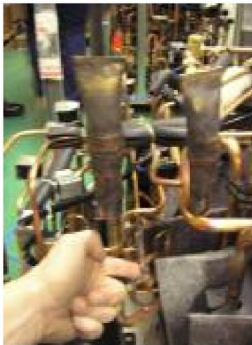
Re-connect the "Hot Gas Injection Circuit"
