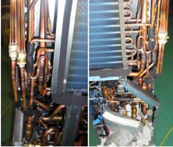
Pipe work after reconnection.
