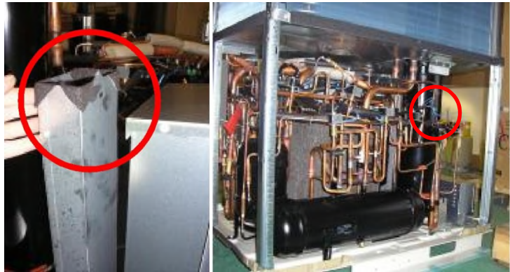
Re-connect the "Hot Gas Injection Circuit"
