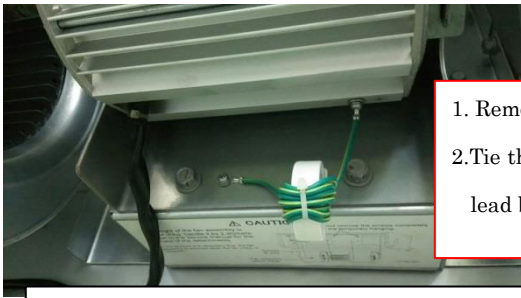
Photo of motor earth lead before repairing
