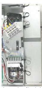
close-up view of terminal block sub-assembly and filter cover
