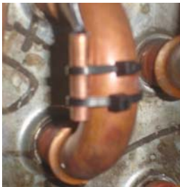
1. Fix to pipe or U bend with two cable ties
