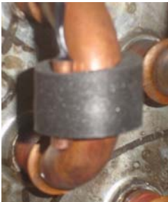
2. Fit the insulation over the sensor
